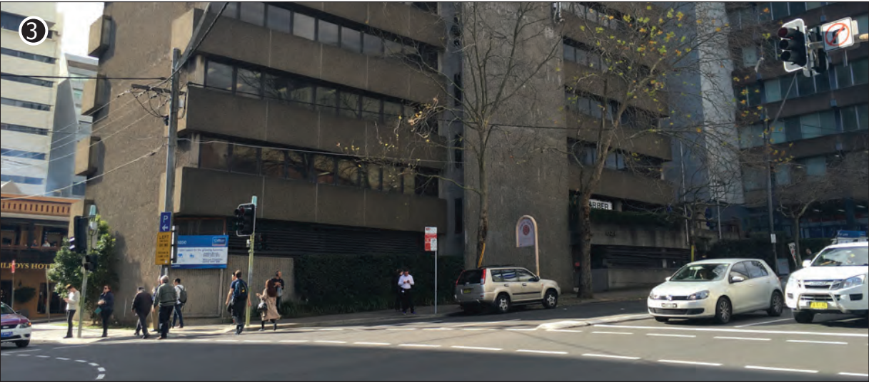
3. View due northeast from the corner of Pacific Highway and Christie Street
