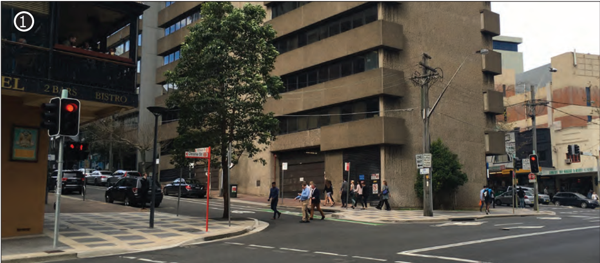
1. View due southeast from the corner of Sergeants Lane and Christie Street
