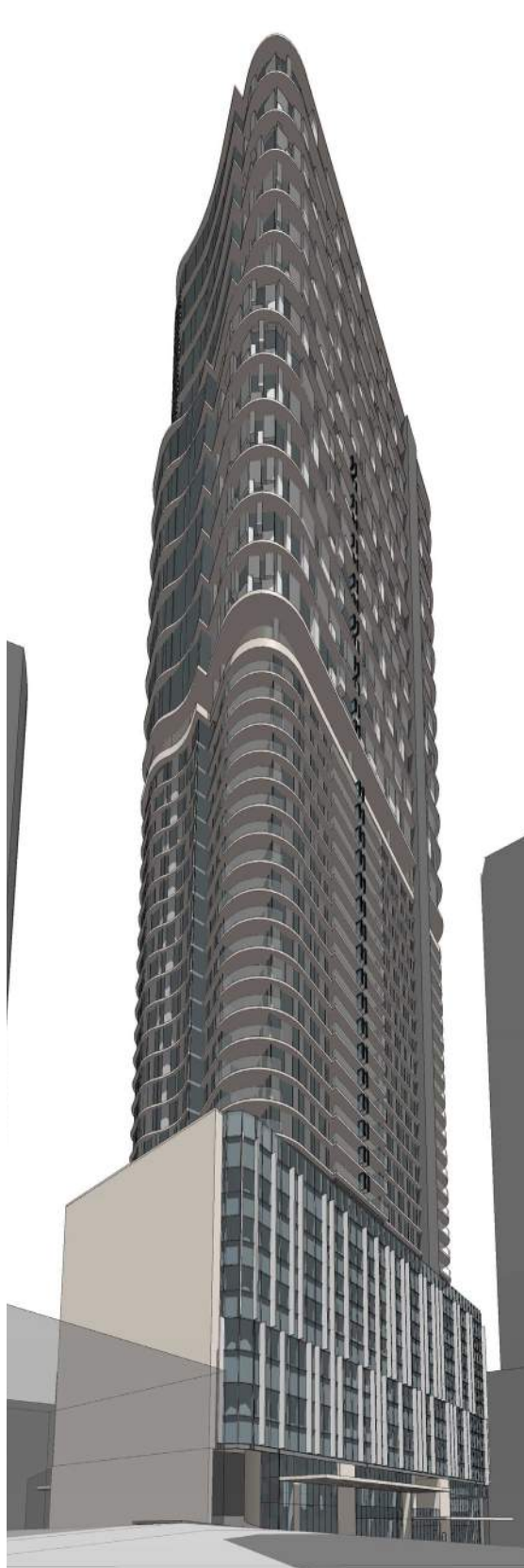
VIEW FROM NORTH EAST
